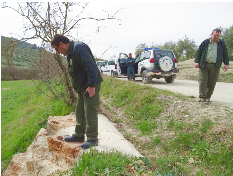
Figure 11. A recent riprap built with Ammonitico Rosso blocks was discovered by the Nature Conservation Police thanks to the orange-red color typical of this lithofacies.
