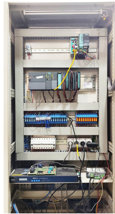
Figure 7. Hardware implementation of the control system.
