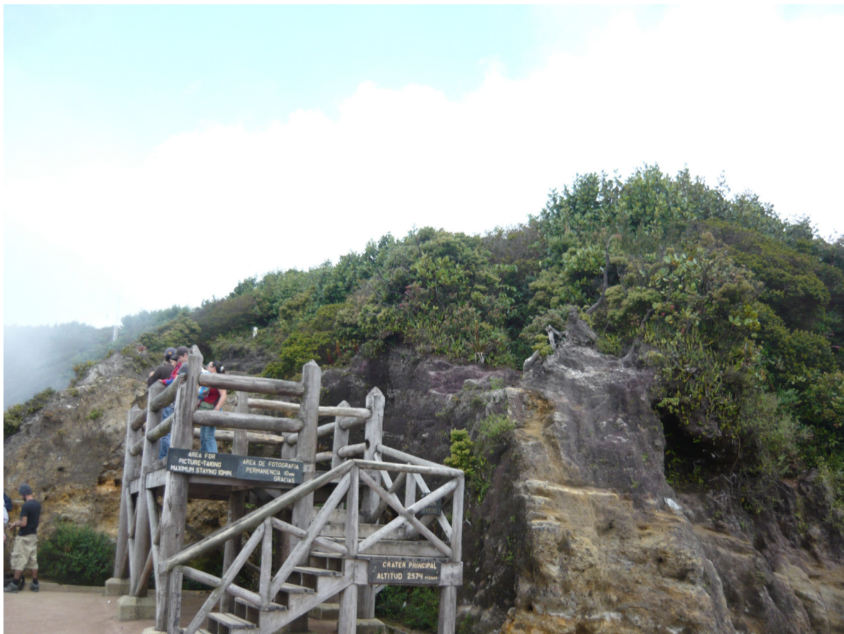
Figure 6. Viewpoint under construction inside the Principal Crater. (Source: Field work).
